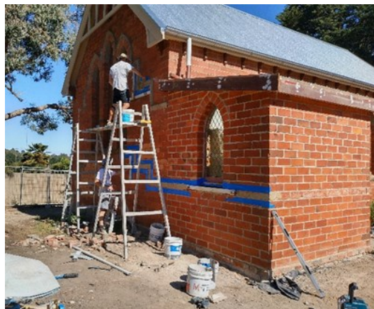
LEFT: New render being applied to the building
